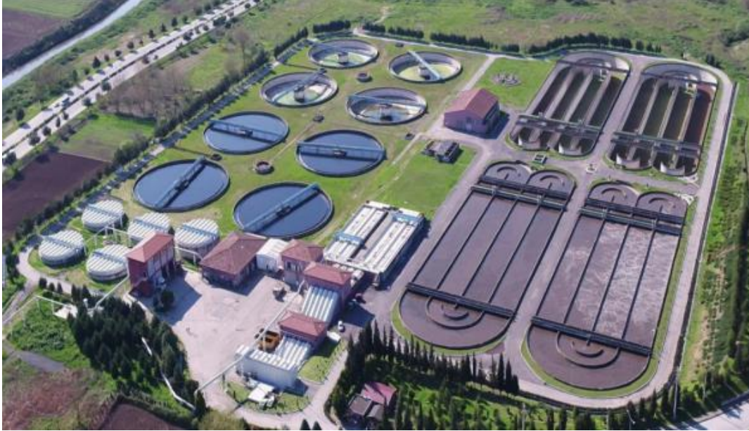
Karaman Wastewater Treatment Facility, Sakarya
