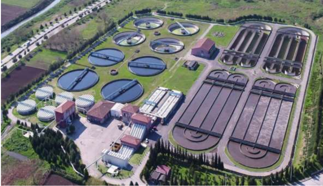
Karaman Wastewater Treatment Facility, Sakarya
